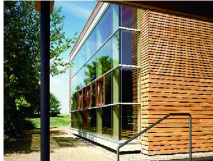
Aula Widukind Gymnasium Enger (1)
